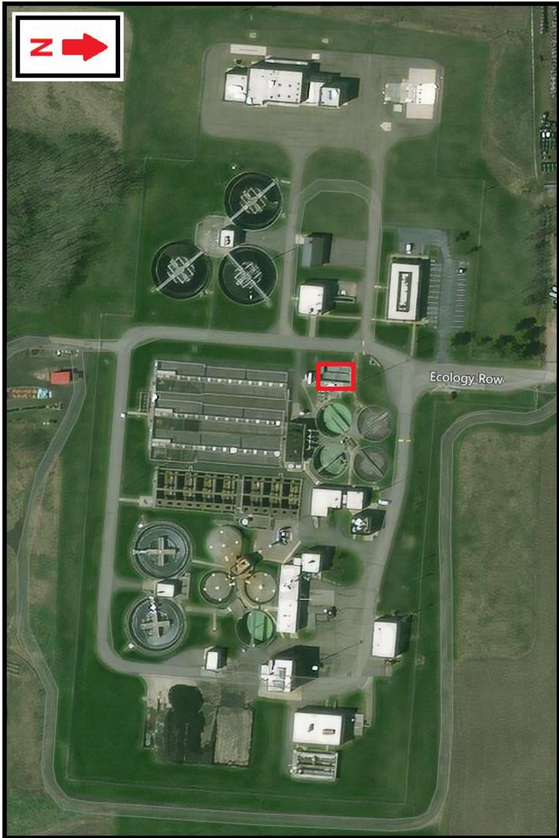
Figure 2. WWTP UV Disinfection Upgrade and SCADA Master Plan project location (in red)
